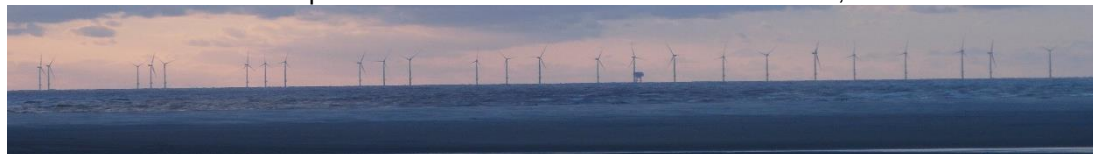
Picture 10 – Wind park Riffgat as seen from Borkum
